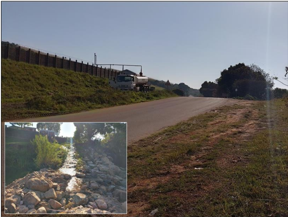
Figure 4-2 Runoff from water truck flowing into river at site Mtwalume US
