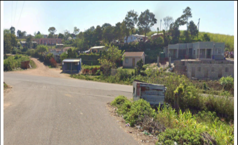
Figure 8: A T junction showing the different roads within the project footprint
