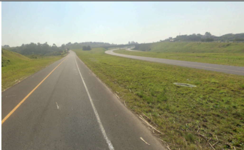
Figure 9:View of the N2 and R102 fly over
