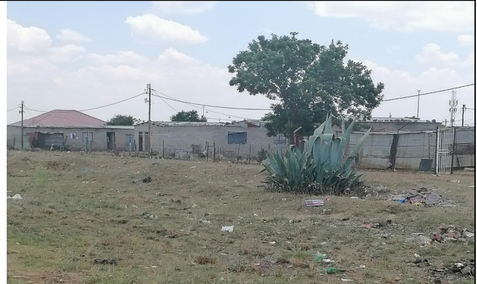
Figure 12: Representational picture of some of the infrastructure in Uswani area
