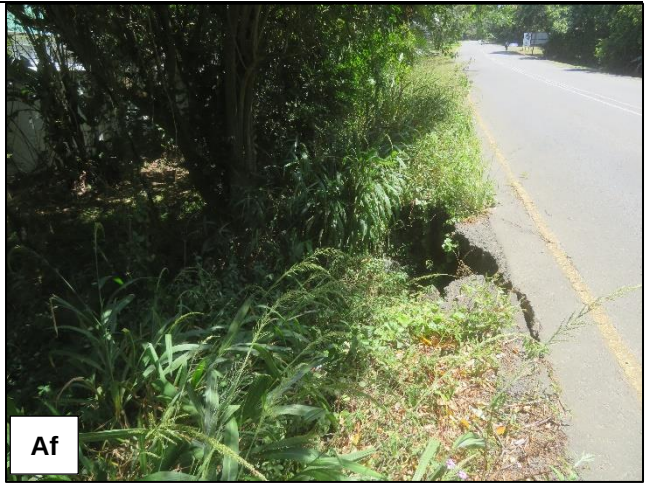
(Ae) View upstream of WC3; (Af) View downstream of WC3, with runoff from the road creating erosion.
