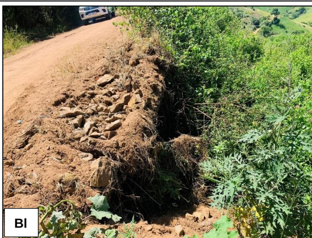
(Bk) Upstream view of WC16; (Bl) Downstream view of WC16, showing erosion on the road caused by water run-off.
