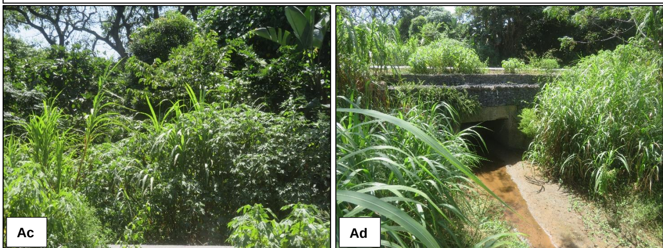
(Ac) View upstream of WC2; (Ad) View downstream of WC2, showing existing culvert structure underneath R102.
